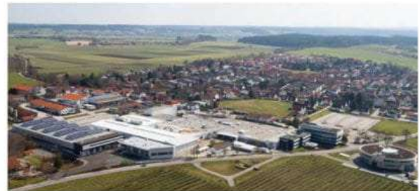
mayr® headquarters in Mauerstetten
